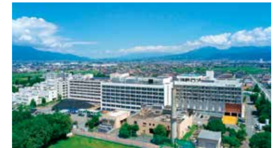
Center photo: New ward Stage II building Right photo: New ward Stage I building
