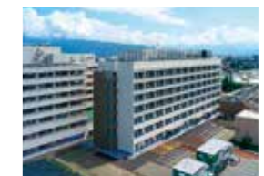
External appearance of New Ward Stage II
